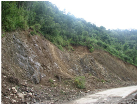
Figure 2 Weak slope material
